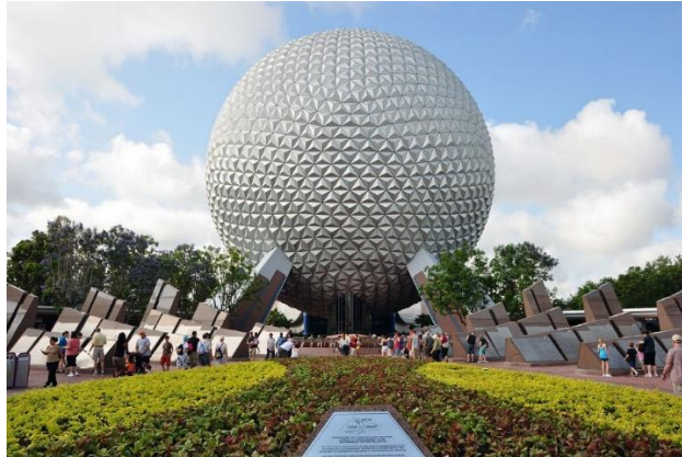
Figure 43: Spaceship Earth structure at Epcot Theme Park
